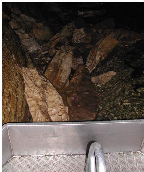
Other pieces of rock in stream bed following scaling. End of the punt in the foreground. Photo: OPUS International
